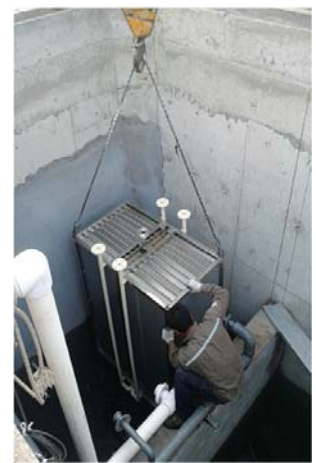
Wastewater treatment MBR membrane module (Taipinggong, Laoshan)
