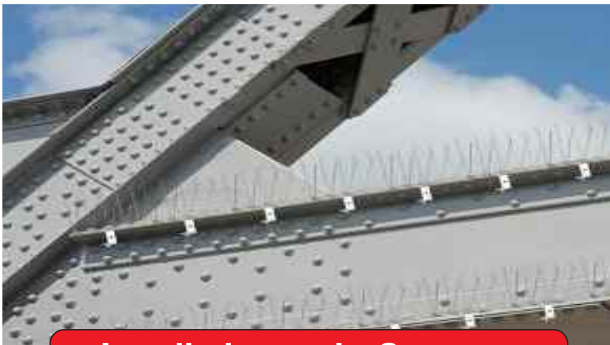
Installation on the Structure
