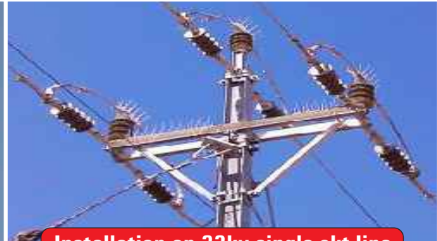
Installation on 33kv single ckt line
