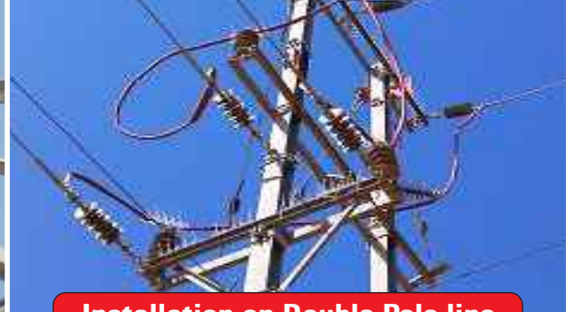
Installation on Double Pole line
