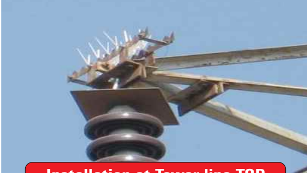
Installation at Tower line TOP
