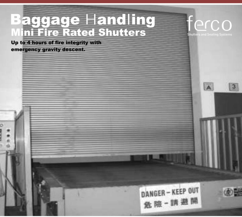
Ferco's Mini Fire Rated Shutters are ideal solutions to enhance security in locations where the opening sizes are small with limited space for headroom and traditional bulky guides.
