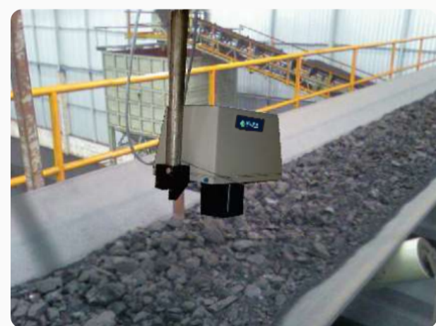
Installation on coke application
