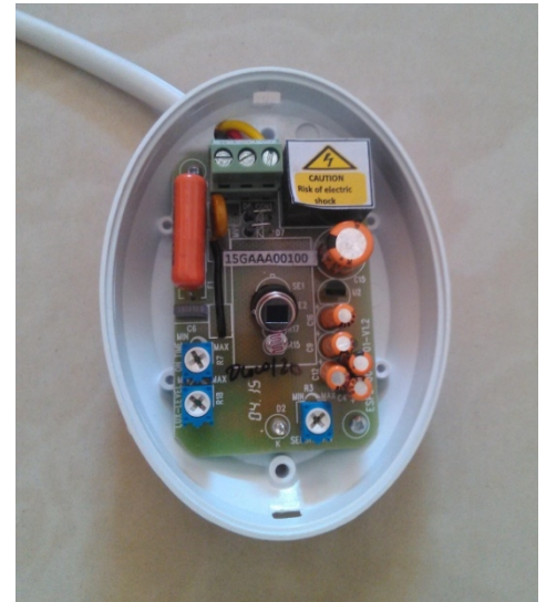
SH02: Inside view
