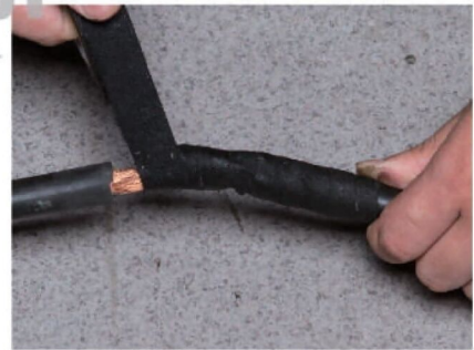
Primary insulation for cable connectors
