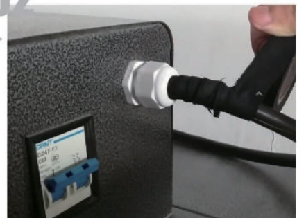
Insulation and repair of cables
