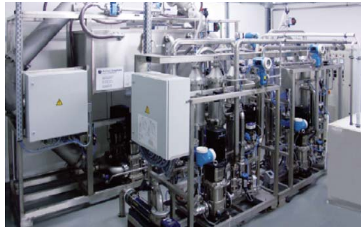
Integrated Ceramic membrane treatment Plant Build
