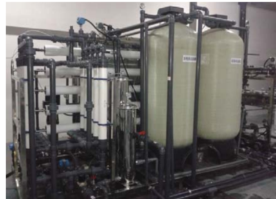
Final RO Plant build
