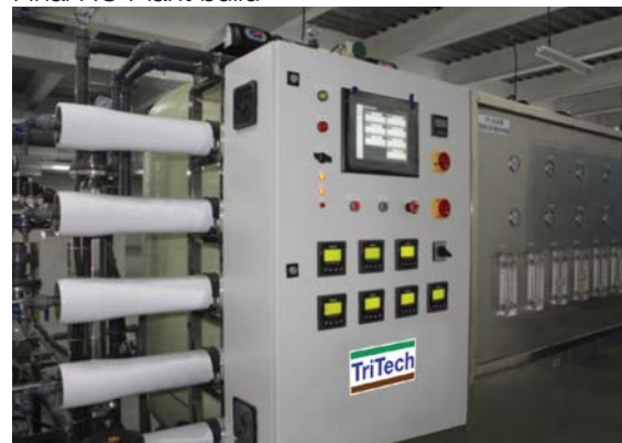
Final RO Plant build
