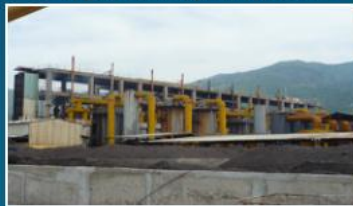
Coal gasification plant, Vietnam
